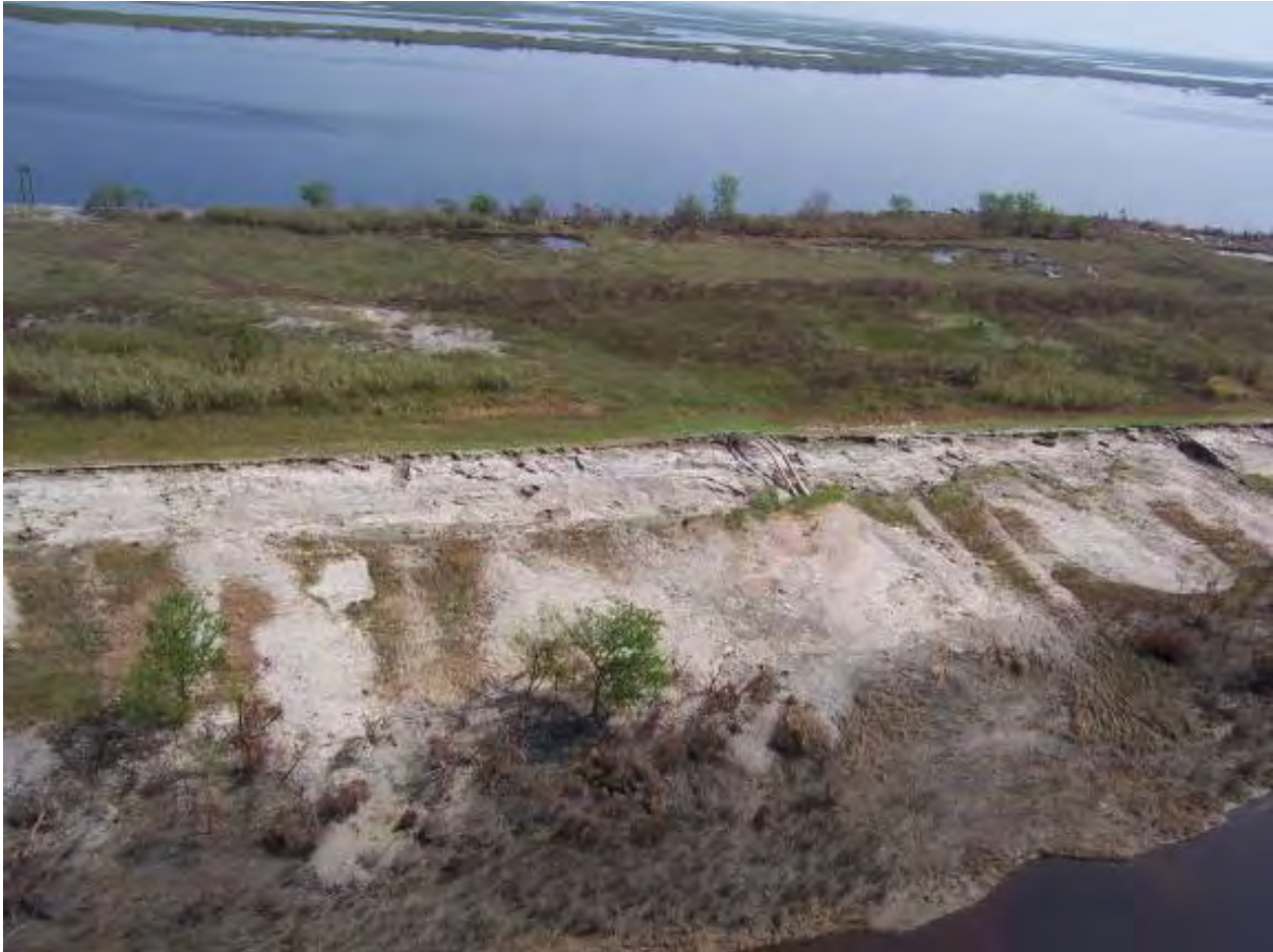
Figure 13-63. 19,000 ft. of Levee Between Bayou Bienvenue (Sta 383+00) and Bayou Dupre (Sta 704+00) Lost Approximately 12' of Levee Height From Original (design) Height 17.5 ft. Pre-Katrina elevation was approximately 12 ft, and storm surge along the MRGO was approximately 18 ft, causing an overtopping crest of up to 6 ft
