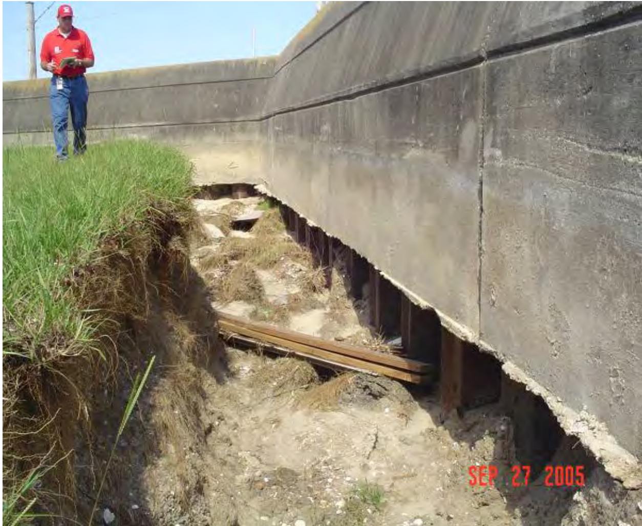
Figure 14-37. Approximate B/L Sta 101+00. Top of I-wall is elev 14.75, bottom of concrete is elev 7, and levee crown is elev 9. Nearest B/L boring is Sta 96+00 (No. 9EU), 500 feet distant
