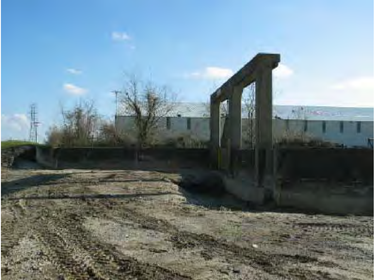
Figure 14-41. Scour at Gate 7E; Scour Measures 7' (w) x 30" (deep). Top of wall is at elev. 13.1 +/-
