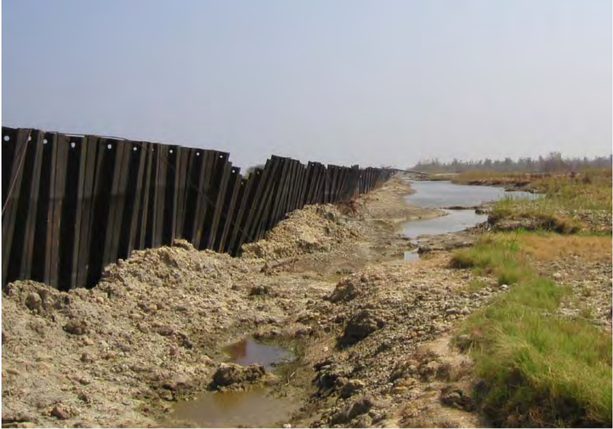
Figure 14-123. Note Sheetpile Elevation Differences
