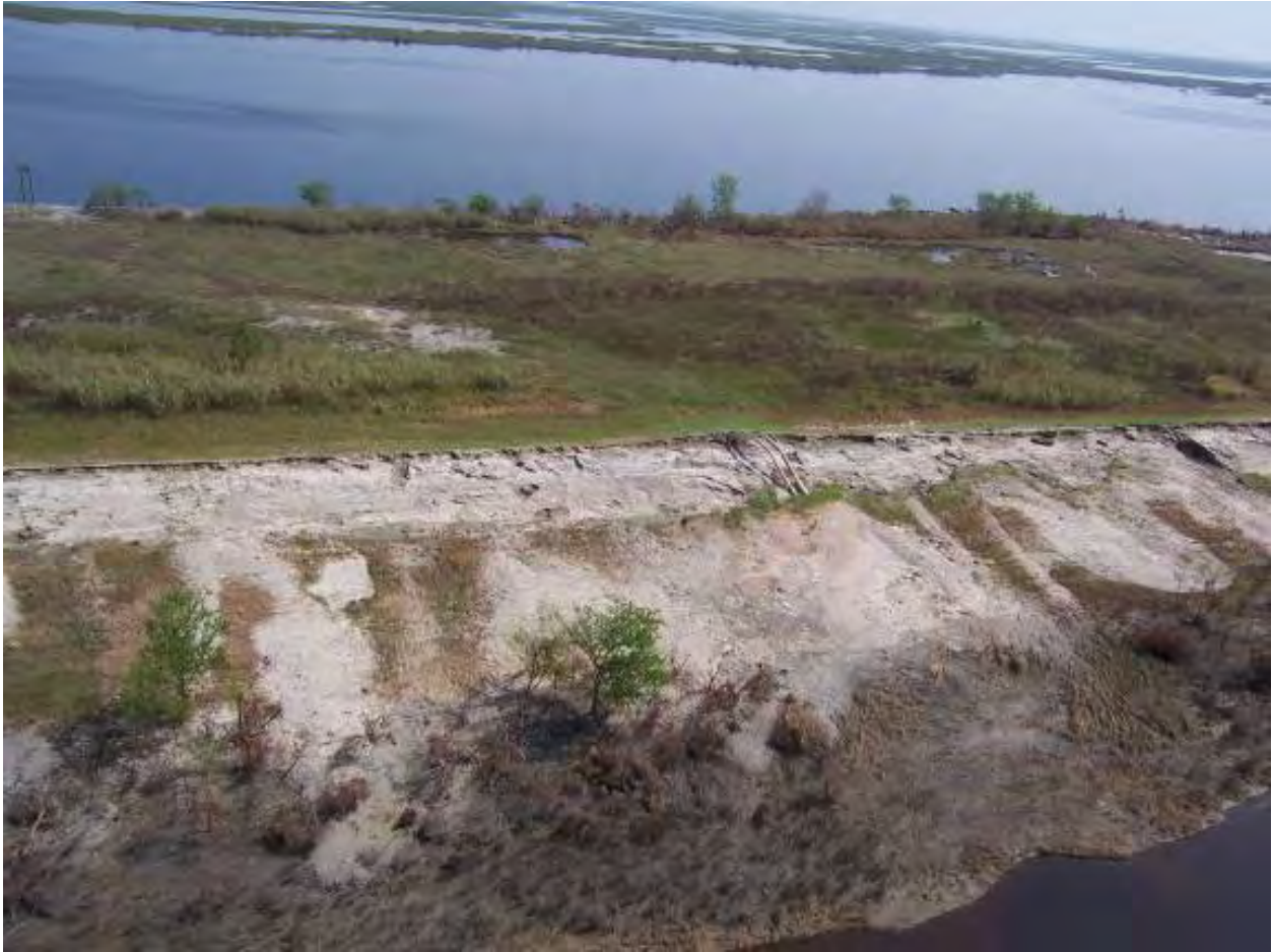
Figure 14-116. Levee Completely Eroded Away
