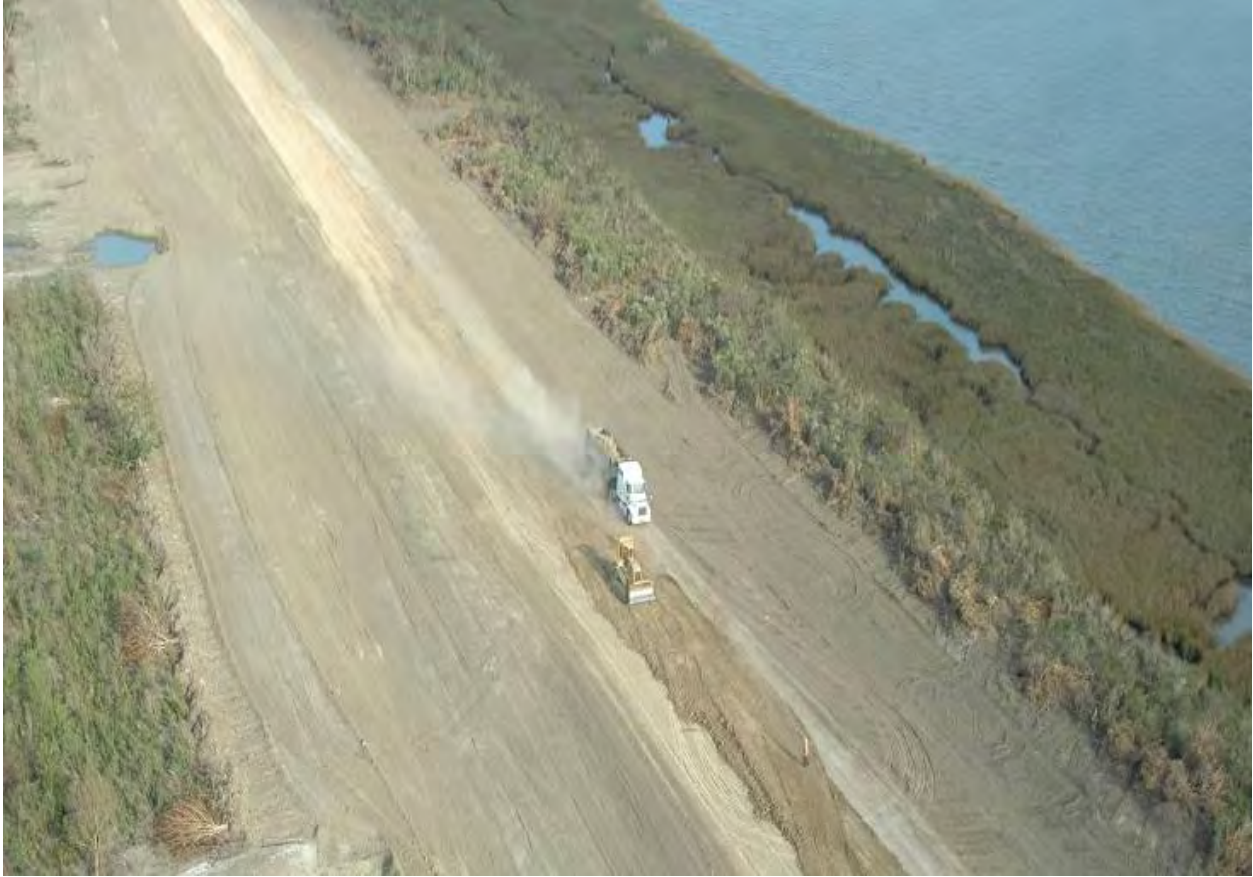
Figure 12-39. NOE1_F Rebuilding to Initial Elevation 10'
