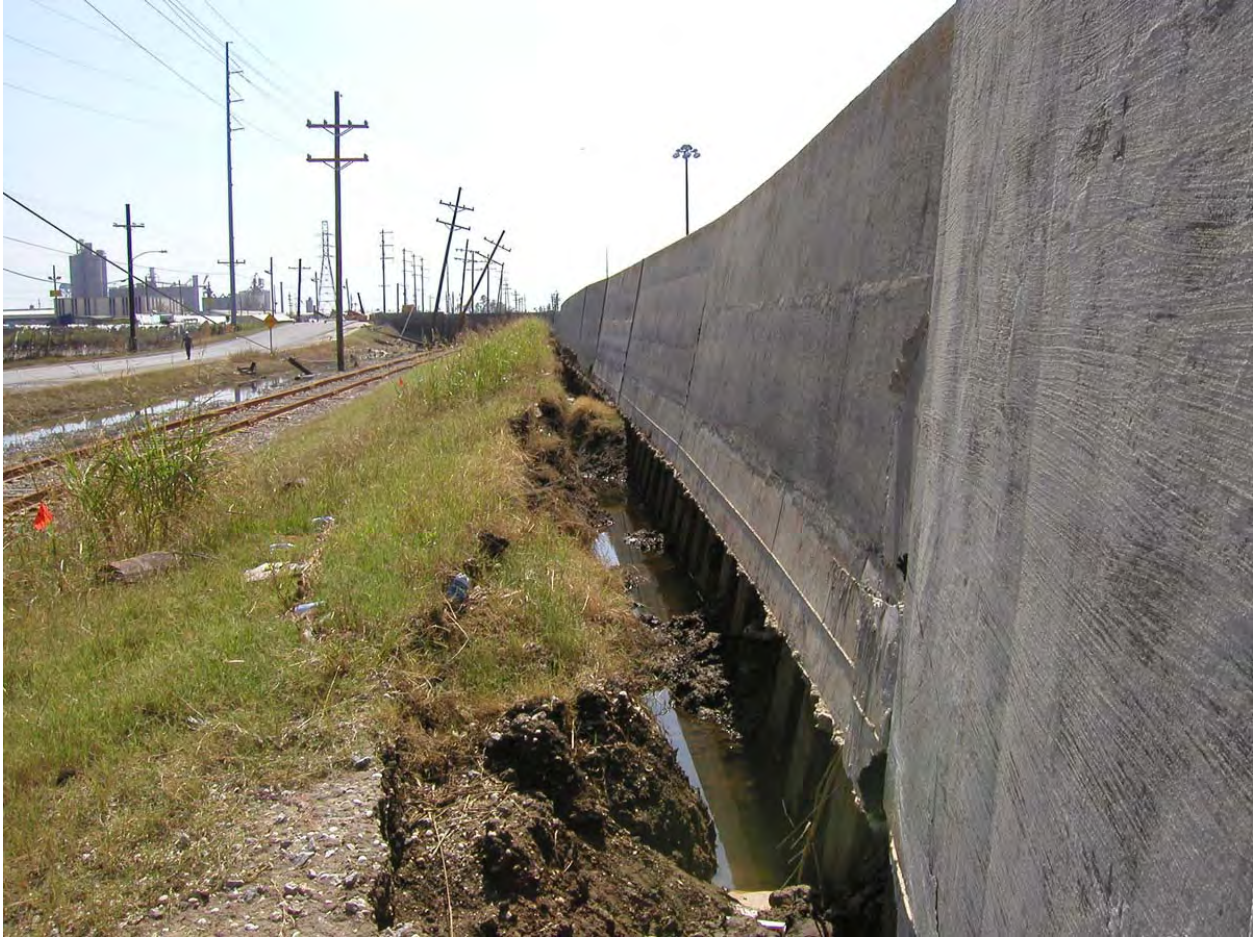
Figure 13-18. IHNC West Side, View South from Benefit St. Gate Toward France Rd Ramp. Approximate W/L Sta 5+56 (B/L Sta 205+44). Top of I-wall elevation 15 ft, levee crown 9 ft, bottom of concrete 7 ft, bottom of pre-existing Z-27 sheet pile (installed by the Orleans Levee Board) at -10ft (MSL). From drawing file H-2-24111, plate IV-15. Nearest soil boring (Figure 13-19) is 30W at B/L Sta 203+00. The I-wall rotated and floodside levee deformation occurred, probably as a result of sheetpile rotation opening up a floodside tension crack. This picture represents scour pattern "C" which is a pre-breaching failure mode
