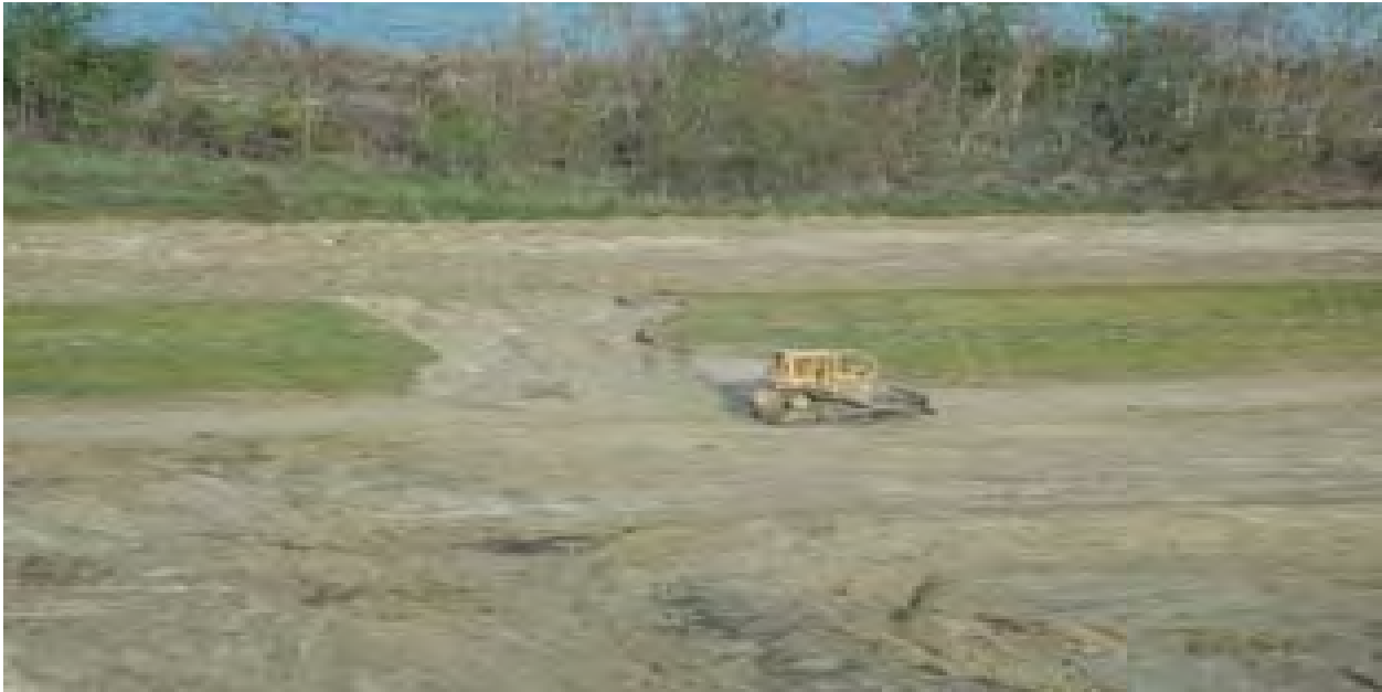
Figure 14-130. Repairs Underway, Filling Scour Holes
