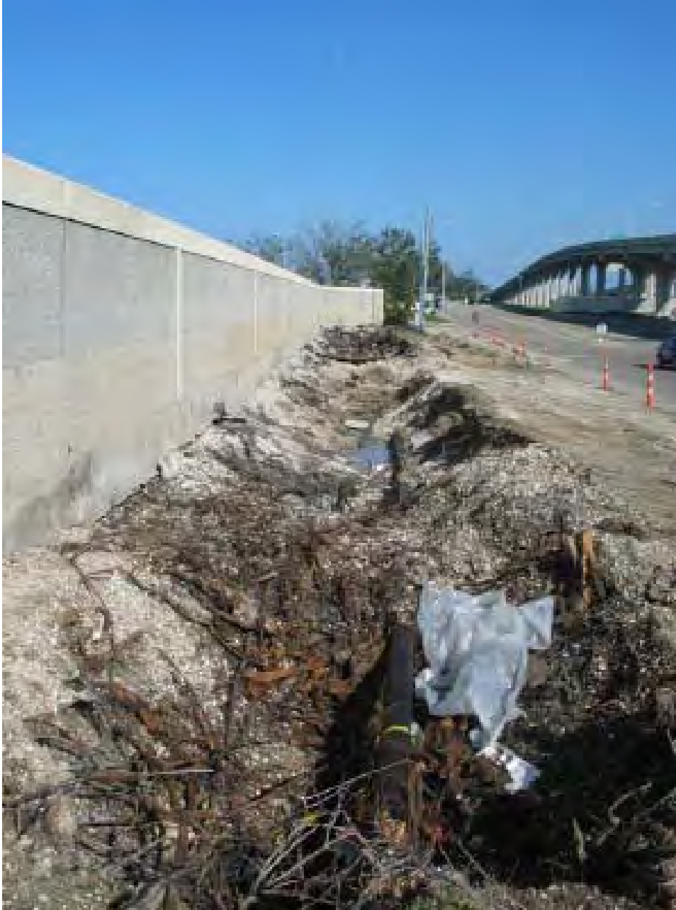
Figure 13-12. Scour Along Lakefront Airport Floodwall Measures 305' (L) x 14' (w) x 48" (d). Existing levee crown appears to be composed of sandy material, based on visual observation. Nearby soil boring 1-C (5/29/1969) at Sta. 8+85, 57 ft right of B/L shows sand, silt, and lean clay lenses to 9-ft depth. Soil boring 4-A (11/3/1970) at Sta 18+00, 200 ft landside of B/L also shows sand, silt, and lean clay lenses to 9-ft depth
