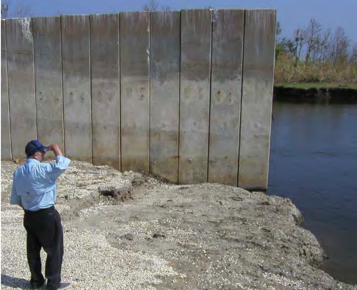
Figure 14-140. Missing Levee and Part of Wall on West Side of Control Structure
